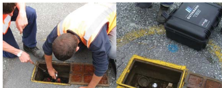
Figure 2: Installing an Acoustic Logger in Queenstown
