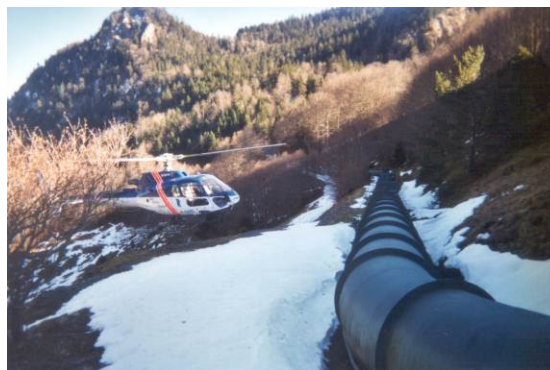
Picture: example of DN 1500 mm pipe flow measurement in France
