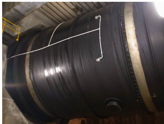
DN 7,400 mm pipe flow measurement in South Africa
